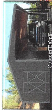
24x36 Barn (12x24 storage; 2 12x12 stalls; 12x24 overhang; stall enclosures and sliders. $20,000 installed)
