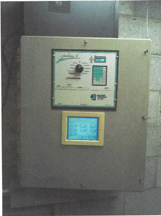
Fig. 1 Existing Items 1 & 2, front
